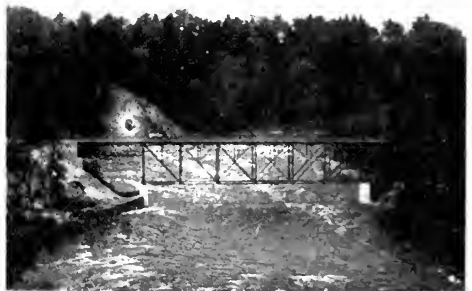
Bridge at Donnacona on the Montreal-Quebec Road. Span, 155 feet between main piers; elevation 50 feet above high water level.
